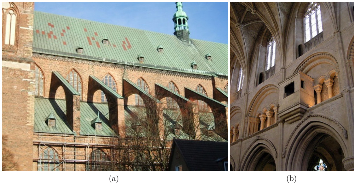
(a) Clerestory between two roofs in St Nicolai Church, Stralsund (left) (b) Clerestory, triforium, and arcade in Malmesbury Abbey, Wiltshire (right)
